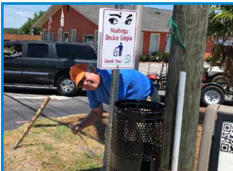
Installation of Pawmetto Pride litter containers on Decker Blvd
