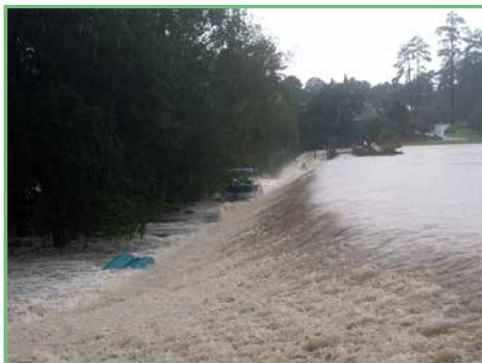
Forest Lake dam overtopped but holding due to armoring, 1pm October 4. Photo Erich Miarka.
