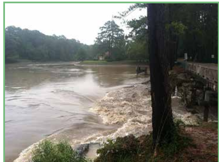
Upper Rockyford Lake dam breaches, 3pm October 5. Photo Erich Miarka.
