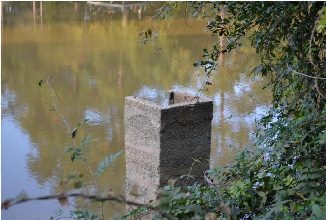
Photo 6: Service spillway drop inlet
