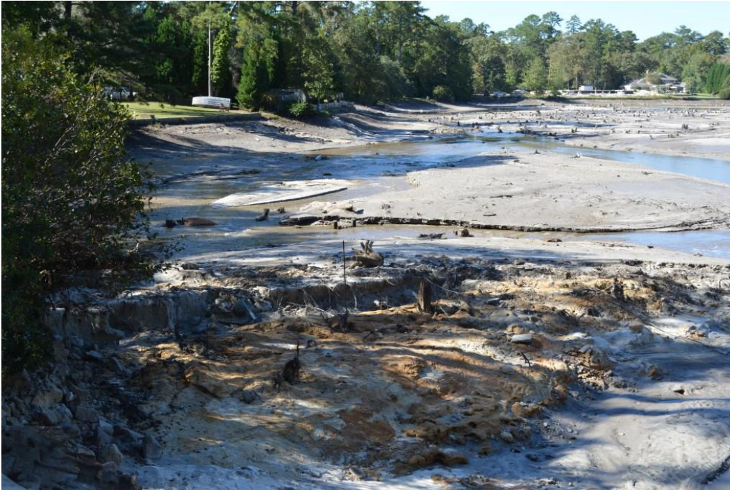
Photo 1: View upstream from the auxiliary spillway
