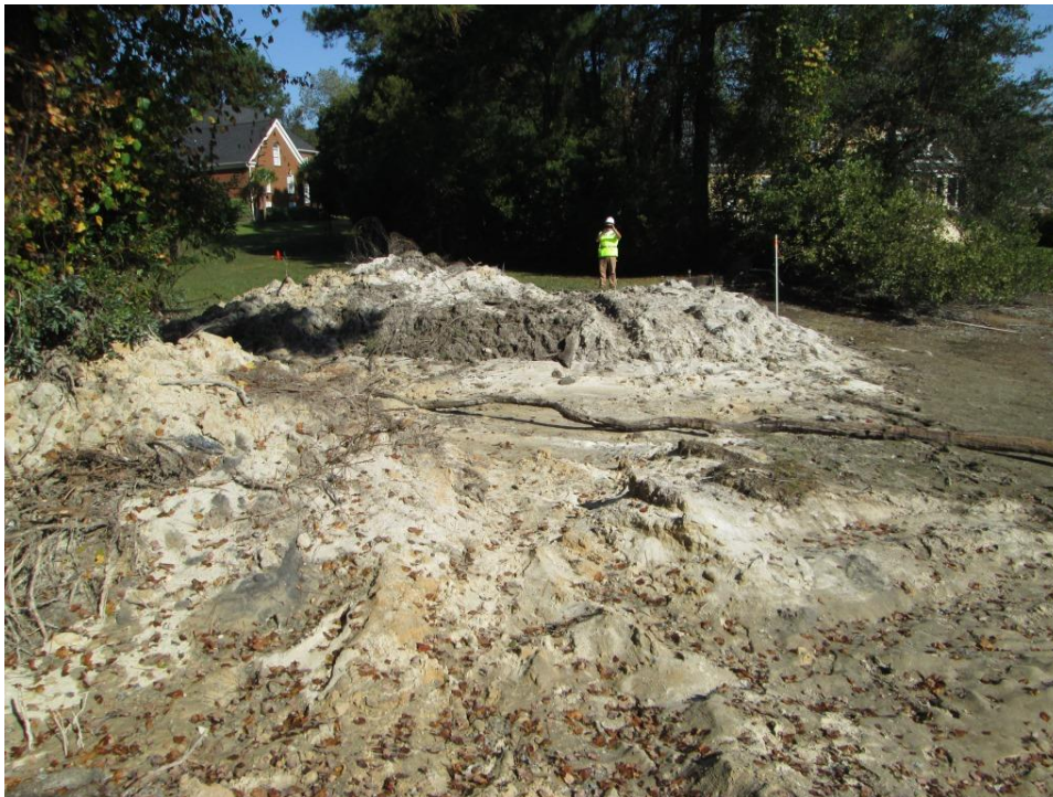
Photo 4: Temporary channel viewed from the embankment
