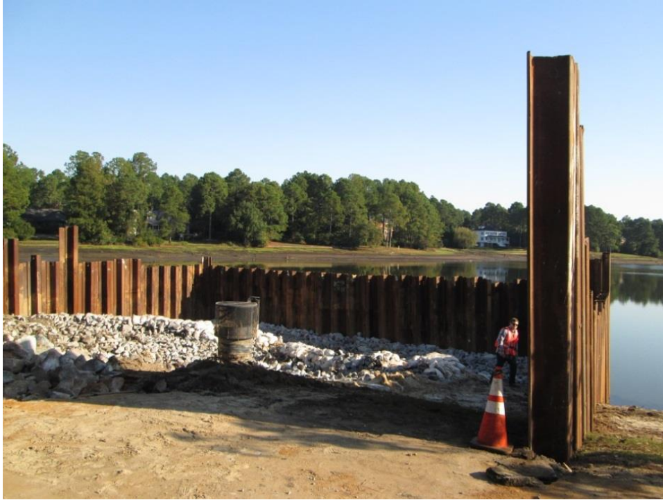
Photo 5: Temporary sheet-pile cofferdam installed to isolate the sinkhole area
