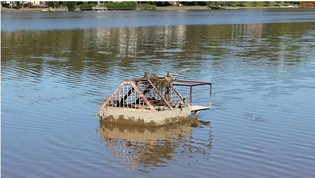
Photo 4: Service spillway concrete riser intake upstream of concrete/rockfill spillway
