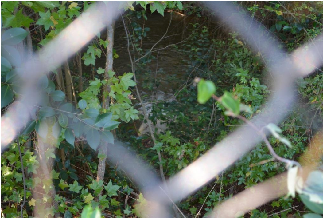
Photo 4: Service spillway outlet pipe
