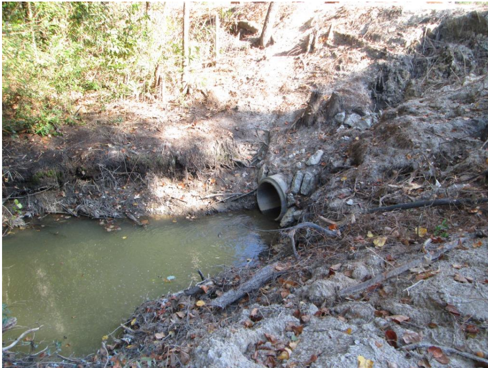
Photo 8: Service spillway outlet
