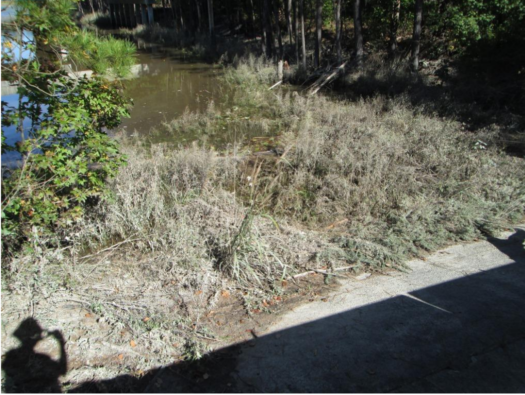
Photo 8: Area upstream of auxiliary spillway
