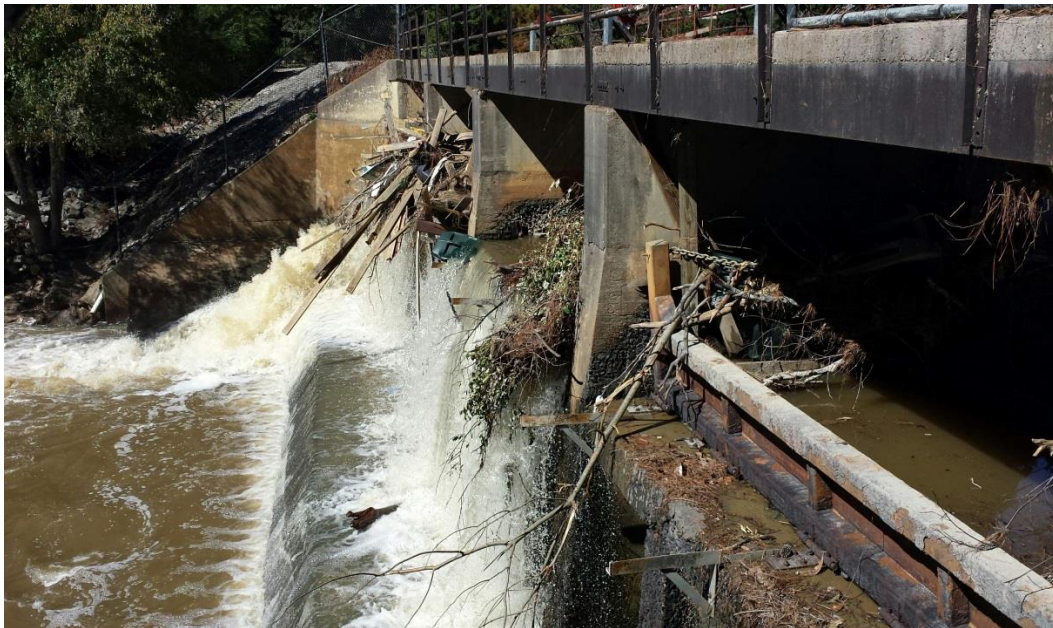
Photo 6: Downstream view of gated, concrete-buttress spillway
