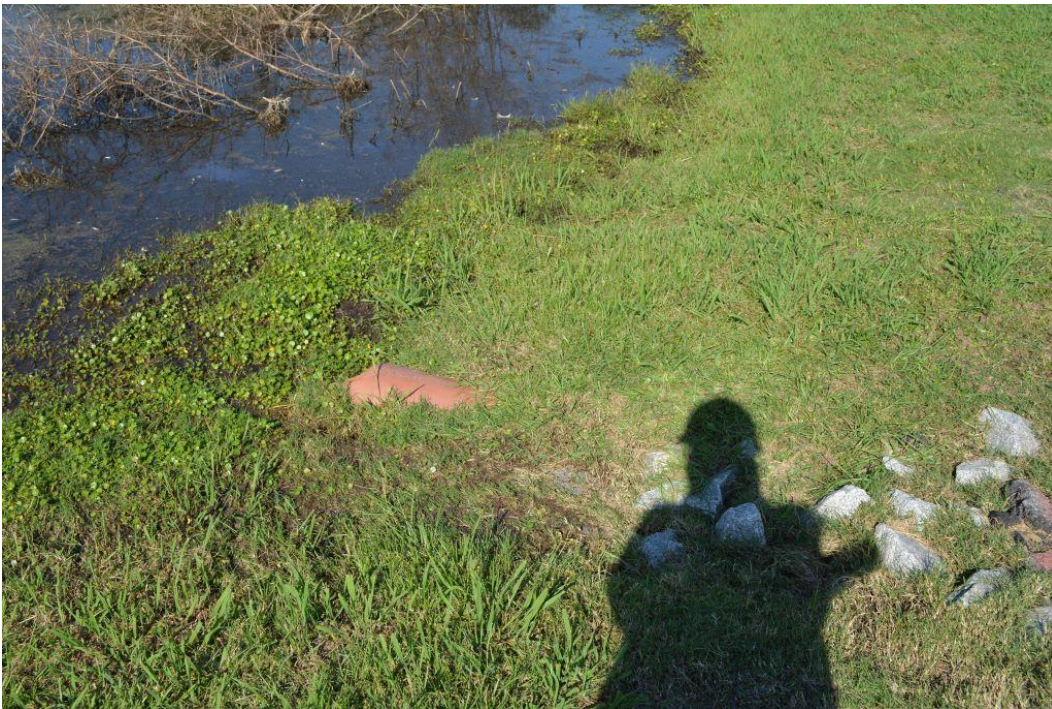
Photo 6: Auxiliary spillway looking upstream
