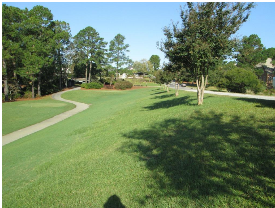
Photo 2: Downstream slope of the embankment dam viewed from left abutment
