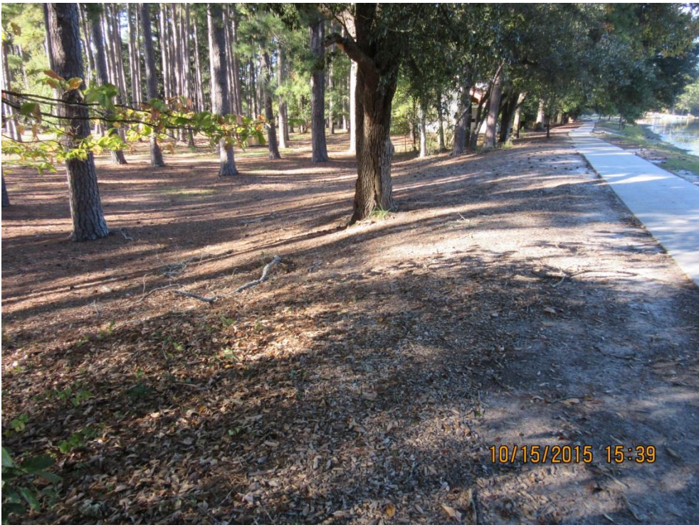
Photo 2: Embankment dam downstream slope and crest with concrete sidewalk
