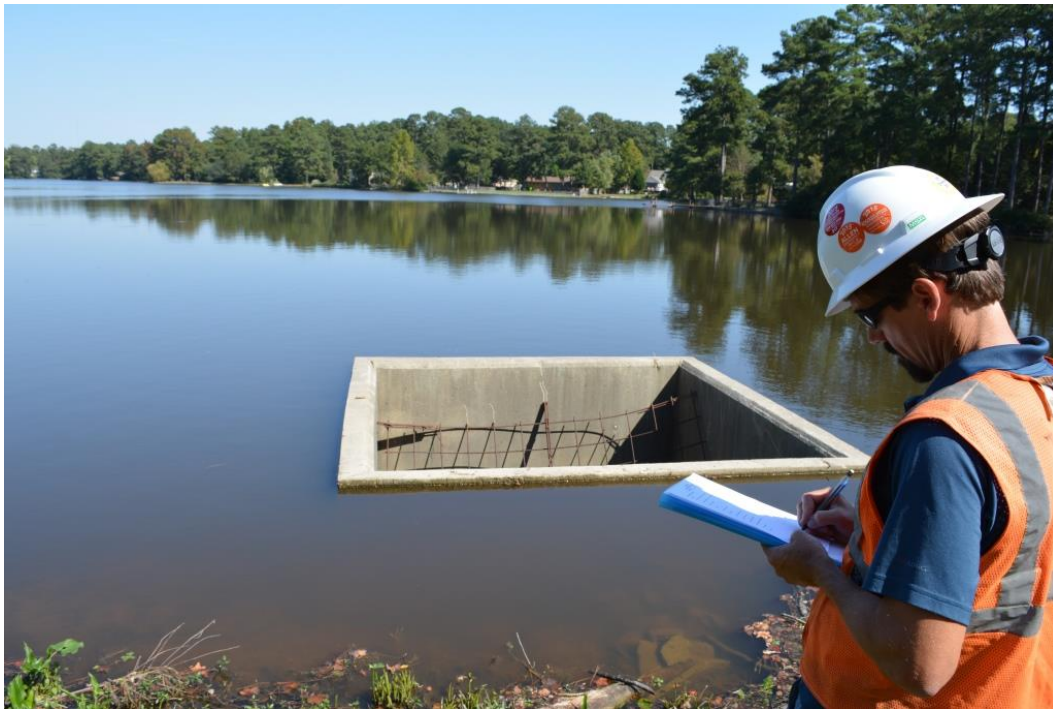
Photo 8: Auxiliary spillway no. 1 intake structure
