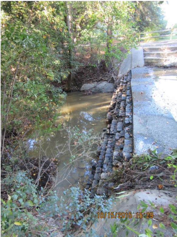
Photo 6: Auxiliary spillway lower masonry stone dam
