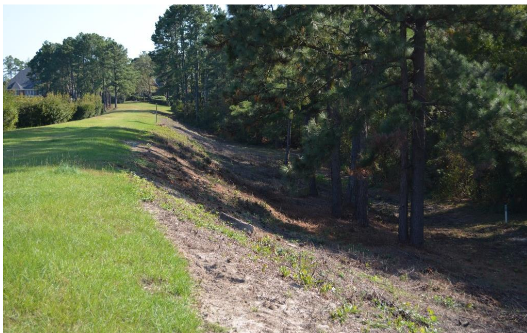
Photo 2: Downstream slope of embankment
