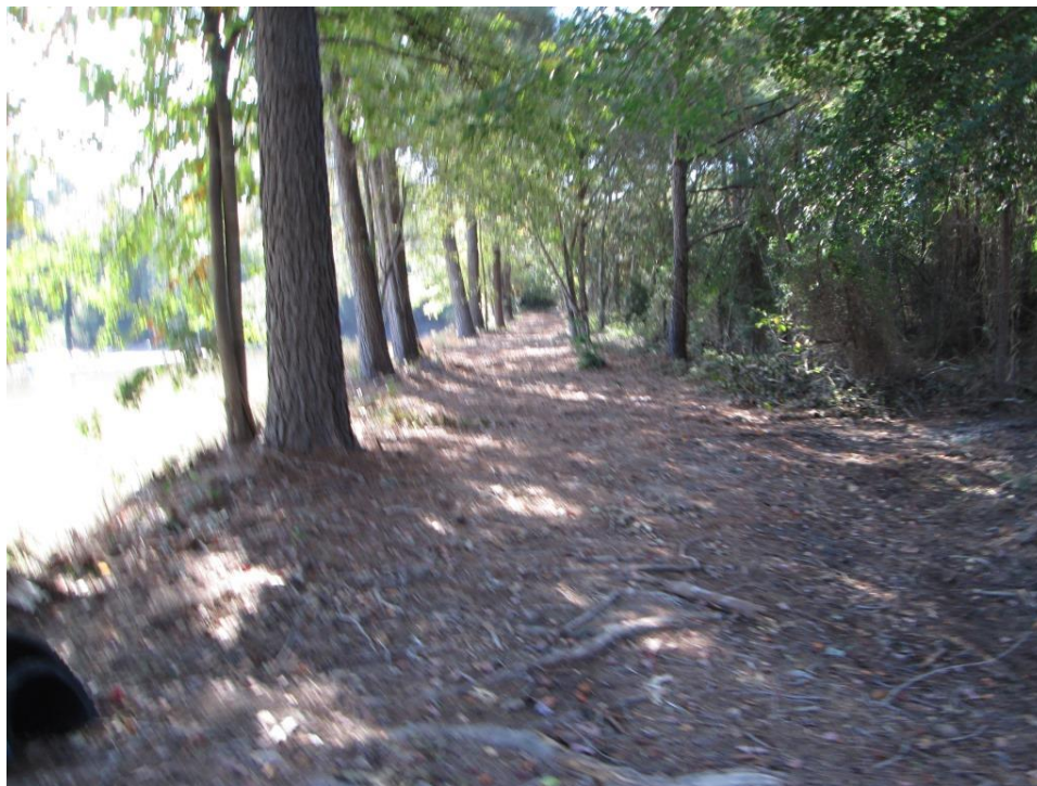
Photo 1: View along crest of embankment dam looking toward the left abutment
