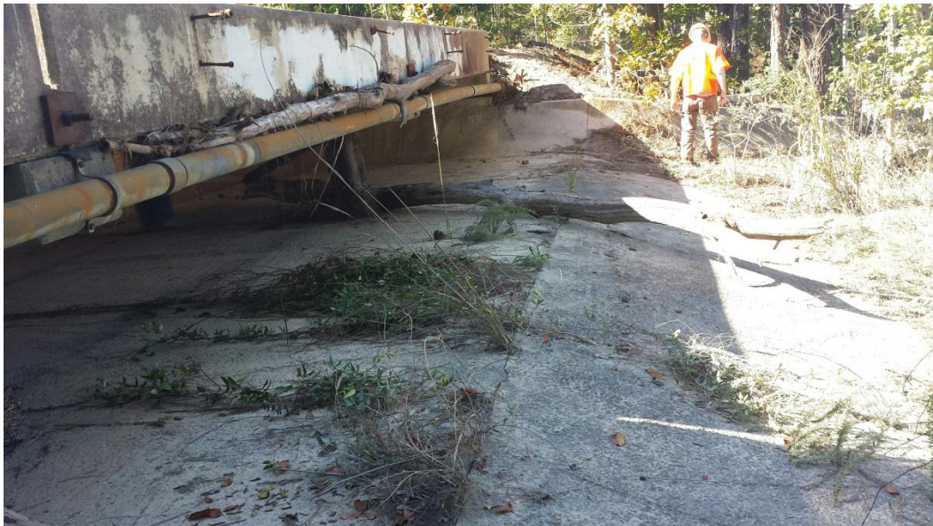
Photo 6: Auxiliary spillway crest looking toward the right abutment
