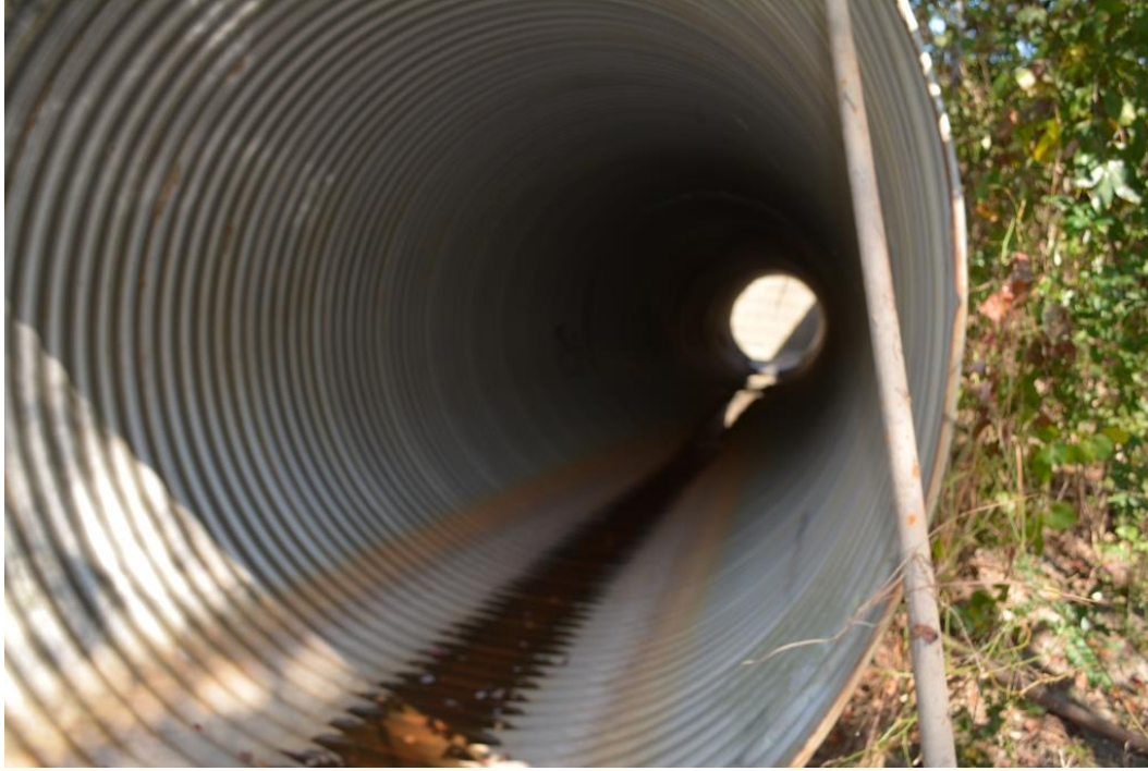
Photo 9: Auxiliary spillway no. 1 pipe (no debris)
