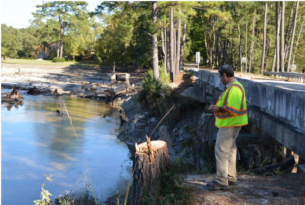
Photo 6: View upstream of bridge and auxiliary spillway
