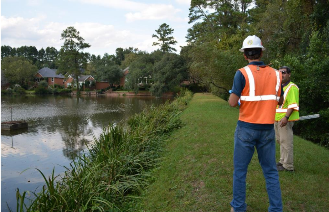
Photo 1: Crest and upstream slope of embankment
