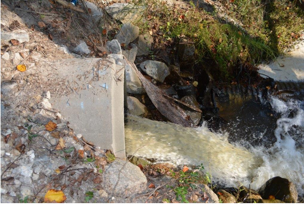
Photo 7: Service spillway outfall
