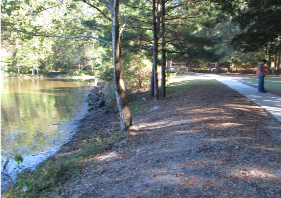
Photo 1: Embankment dam upstream slope and crest with concrete sidewalk
