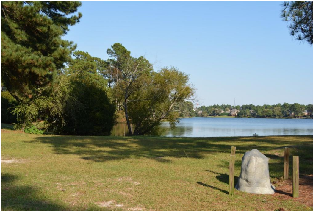
Photo 8: View of auxiliary spillway looking upstream
