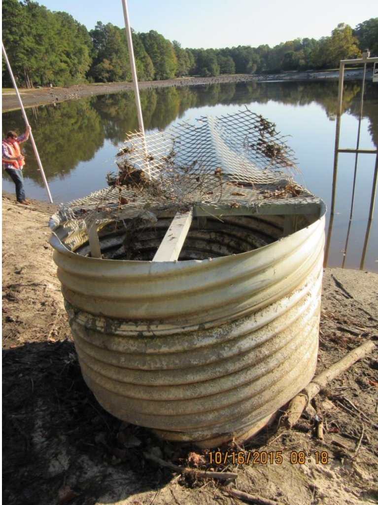
Photo 5: Service spillway drop inlet
