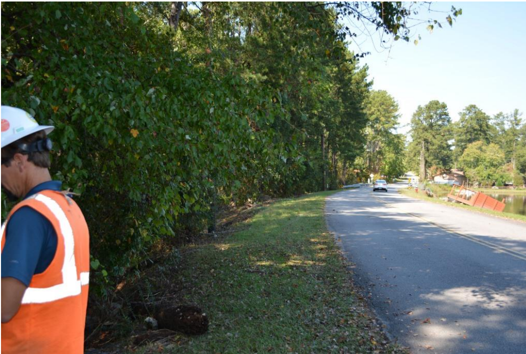
Photo 2: Embankment crest and downstream slope
