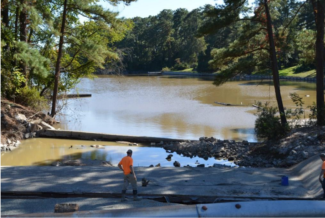
Photo 9: Downstream view from bridge over auxiliary spillway
