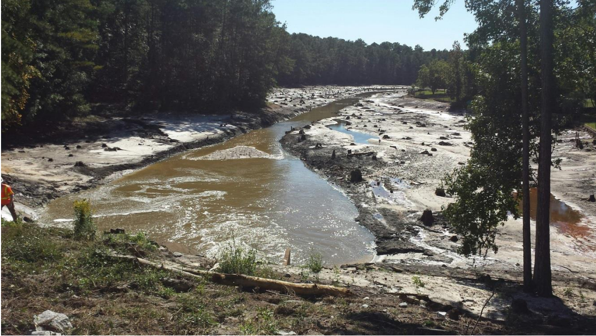
Photo 11: View looking downstream of the dam (Pine Tree Dam, an unregulated dam that breached, is located downstream beyond the bend).
