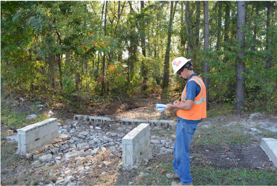
Photo 8: Auxiliary spillway view looking downstream
