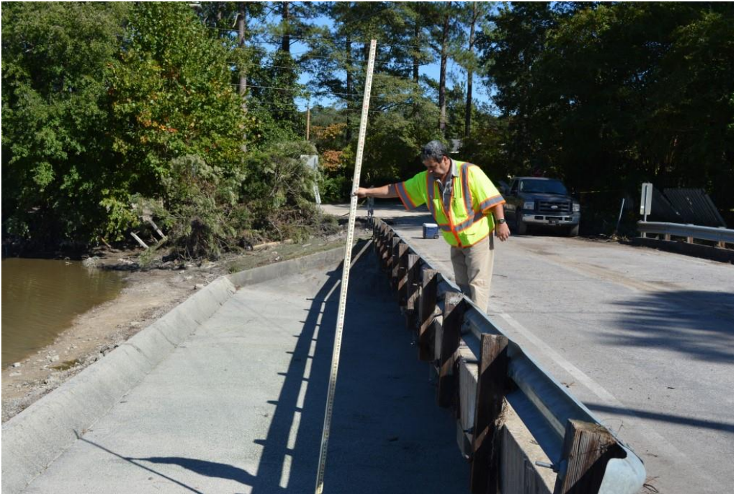
Photo 10: View of auxiliary spillway upstream of bridge
