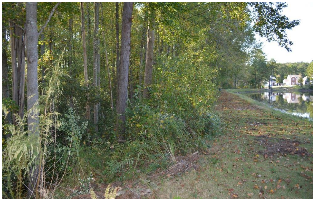
Photo 2: Vegetation along downstream embankment slope
