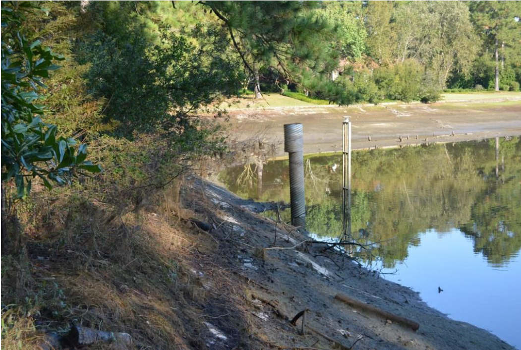
Photo 1: Upstream slope and service spillway intake
