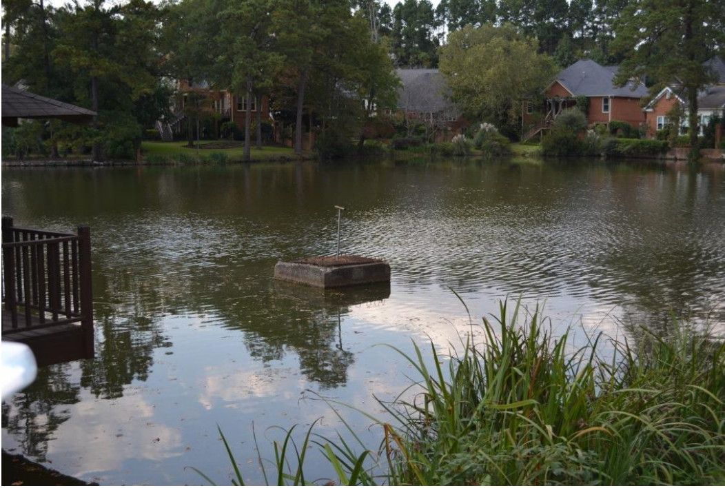
Photo 5: Service spillway intake
