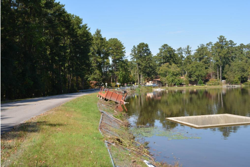
Photo 1: Springwood Lake Dam crest and upstream slope viewed from left abutment
