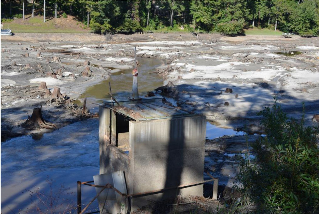
Photo 1: Service spillway drop inlet structure
