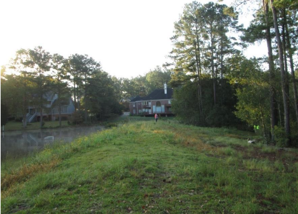
Photo 1: Embankment crest viewed from right abutment. Grass cover on upstream slope; trees and underbrush on downstream slope and toe.
