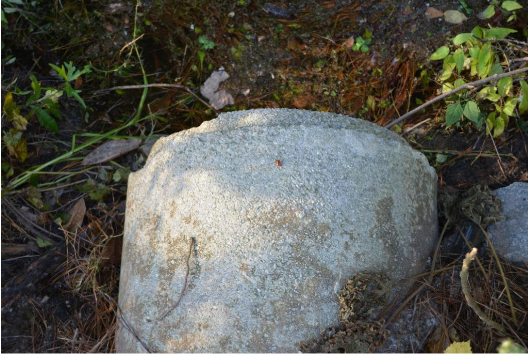
Photo 7: Service spillway outlet
