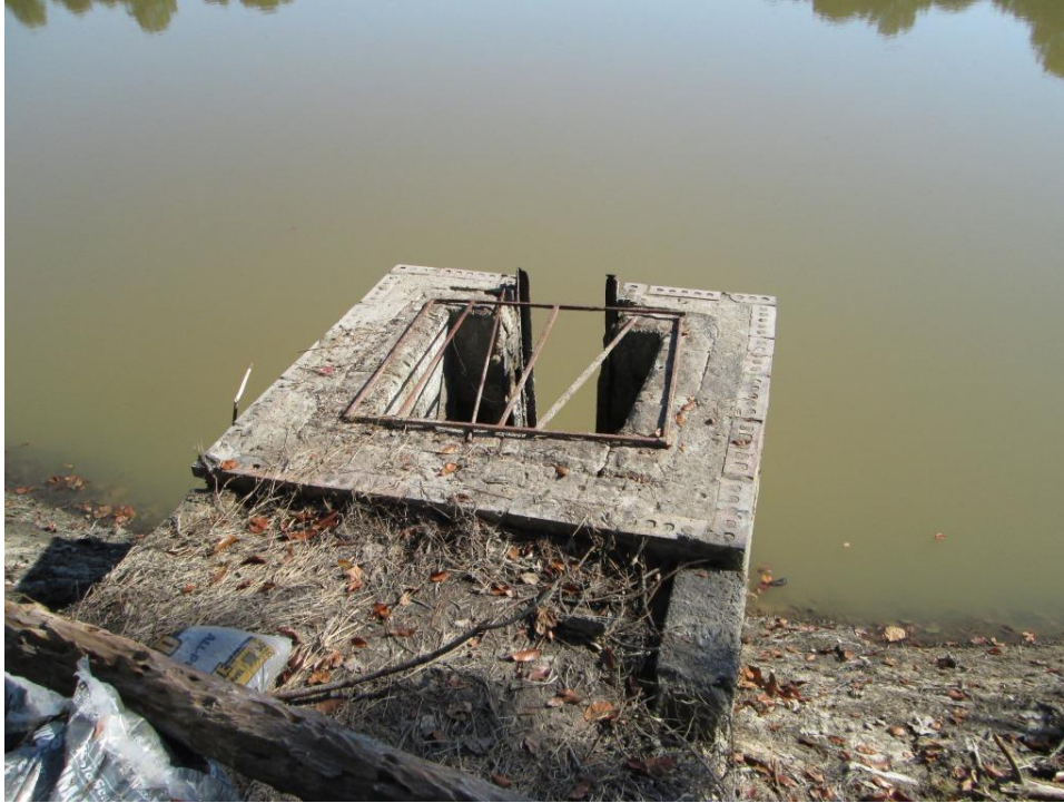
Photo 7: Service spillway drop inlet
