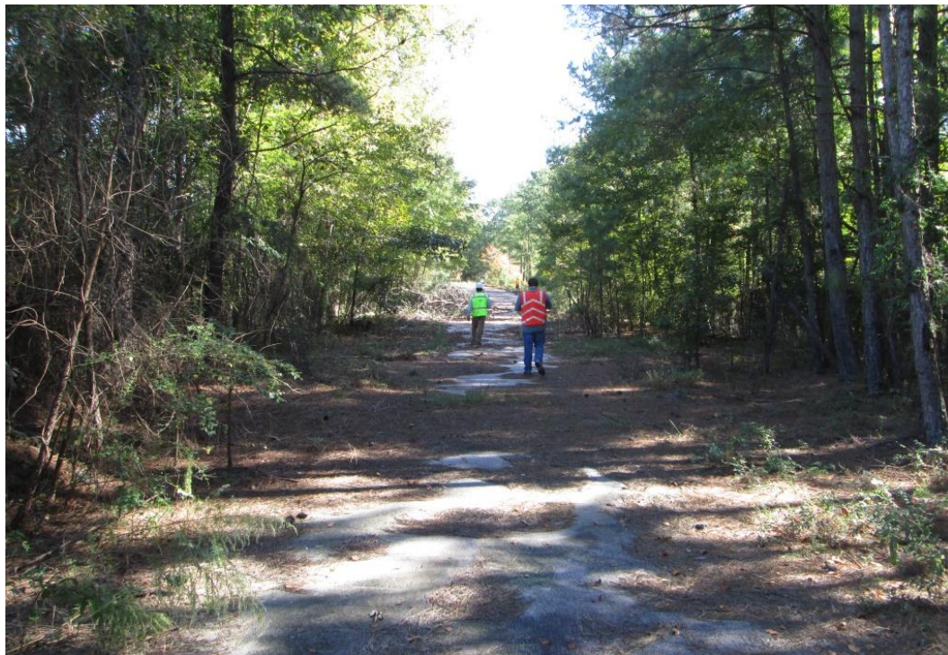
Photo 1: Crest of embankment dam looking toward the left abutment. Note mature trees and thick underbrush on embankment slopes.
