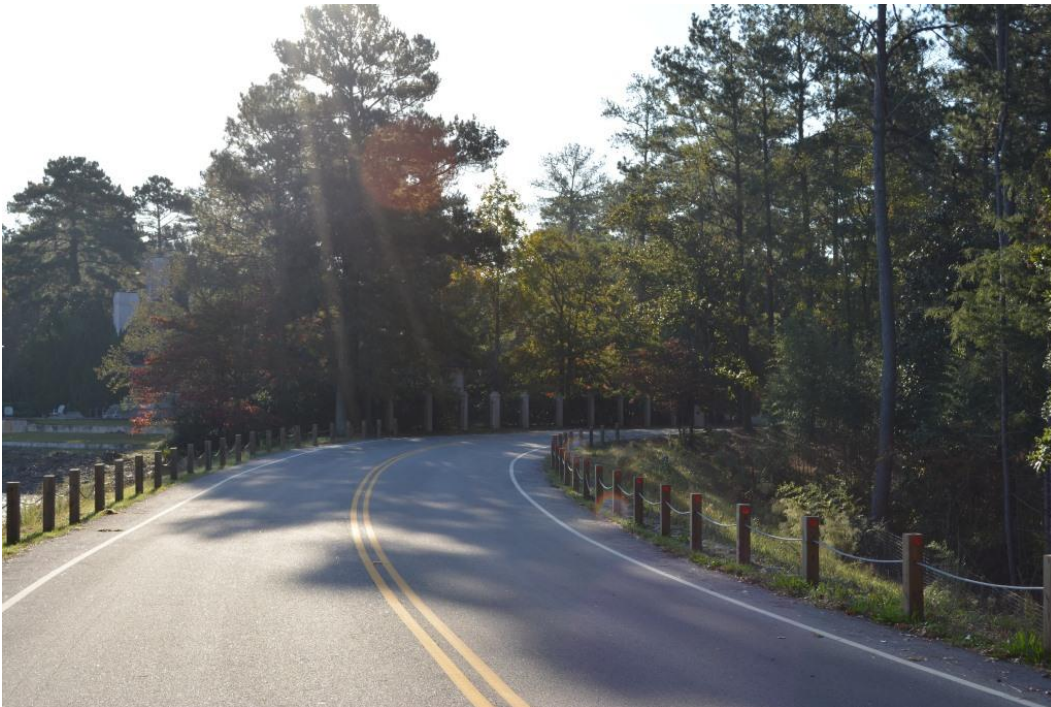
Photo 2: Roadway on embankment crest
