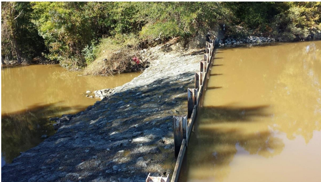
Photo 6: Concrete/rockfill overflow spillway with flashboards
