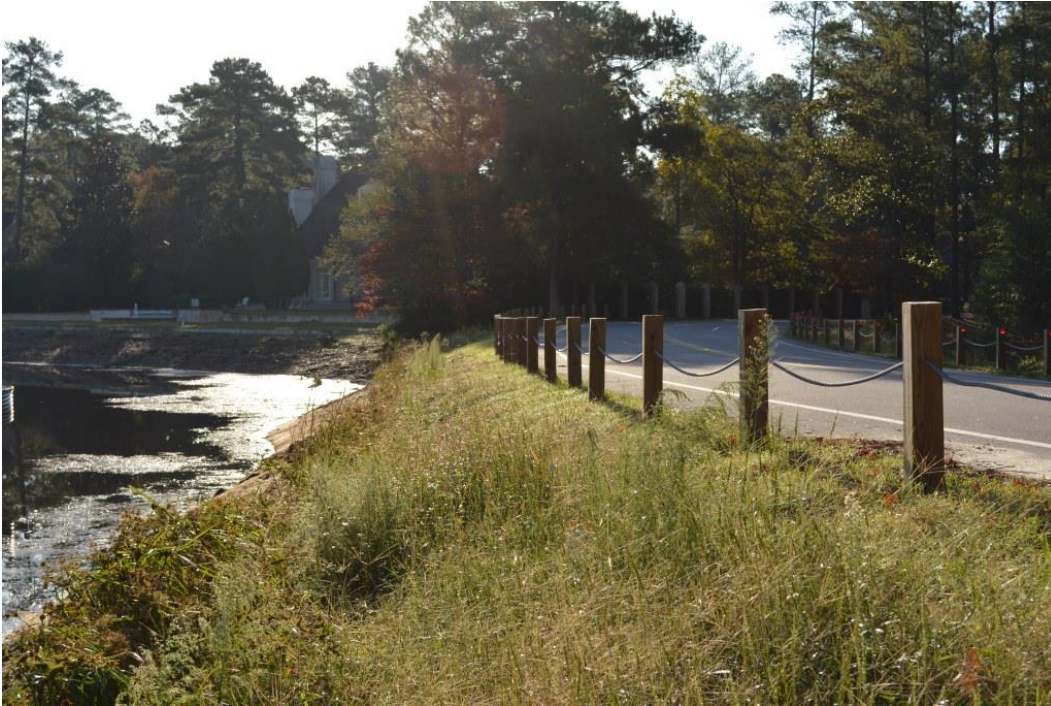
Photo 1: Upstream embankment slope
