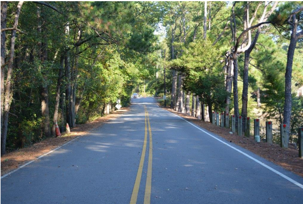
Photo 2: Roadway along embankment crest
