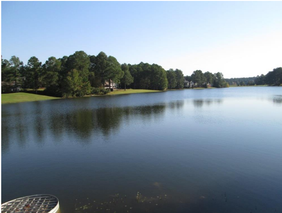
Photo 4: View of pond with service spillway drop inlet in foreground
