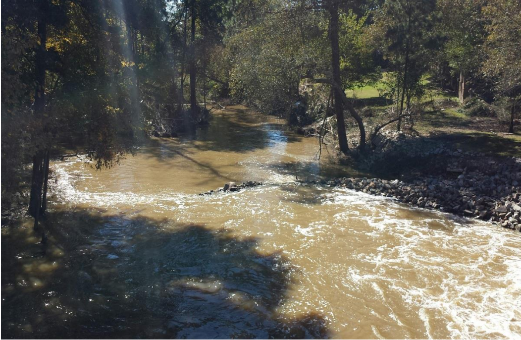
Photo 3: View of downstream channel with rock deposition and riprap on right bank
