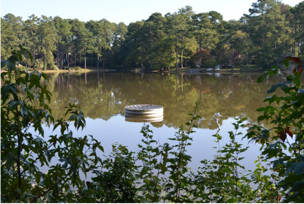
Photo 3: Service spillway intake
