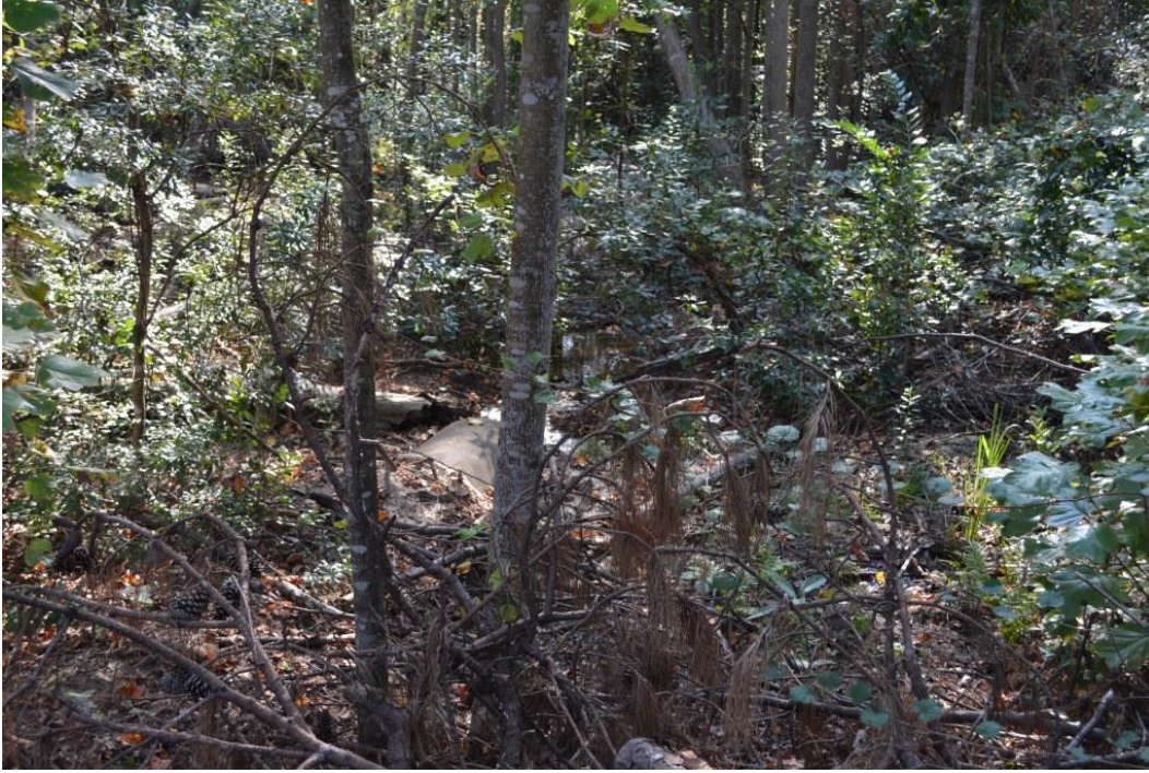
Photo 7: Service spillway outfall
