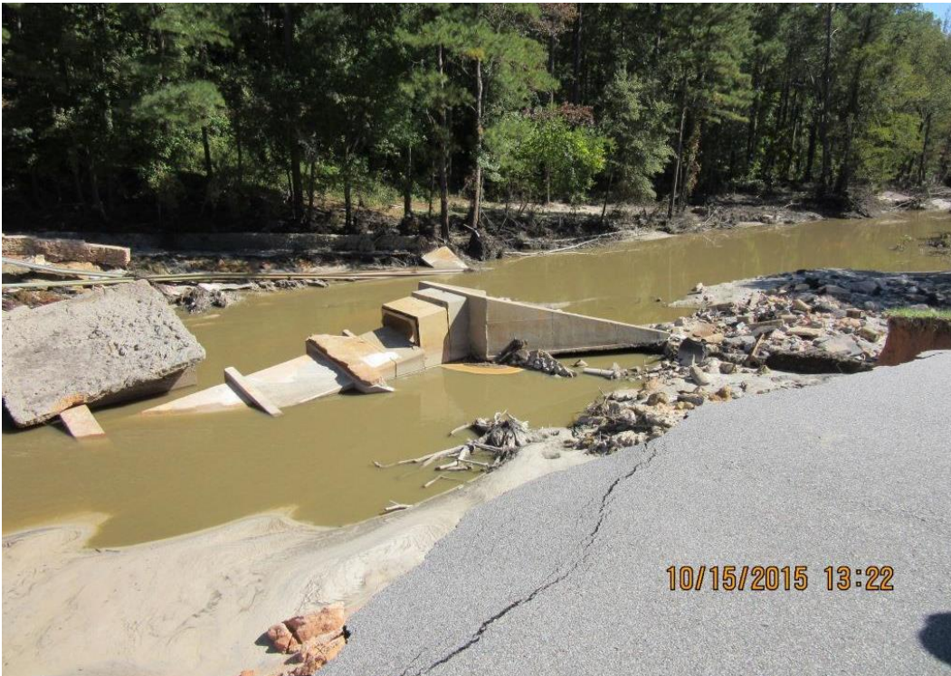
Photo 2: Remnants of low-level outlet concrete box culvert and discharge structure.
