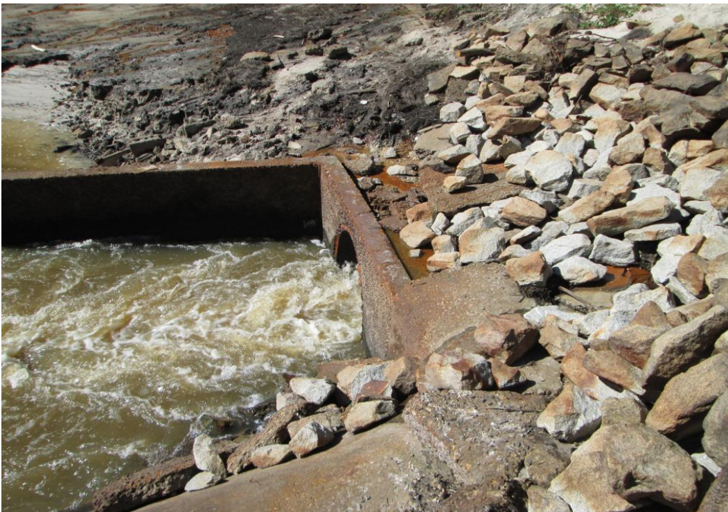
Photo 10: Low-level outlet structure; note discolored water just above the headwall
