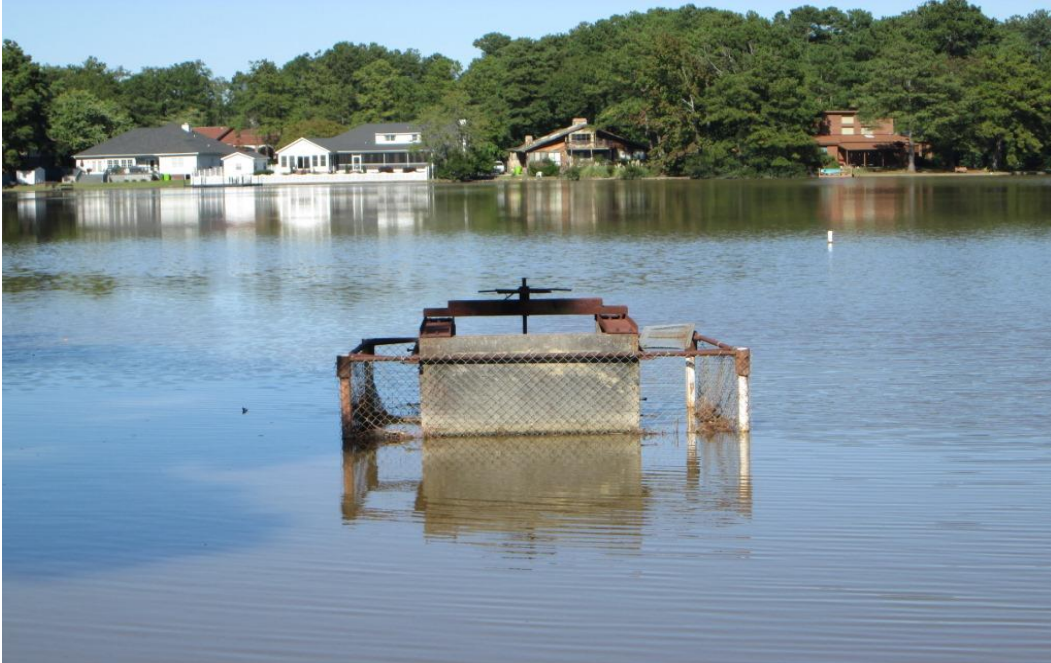
Photo 9: Service spillway drop inlet structure
