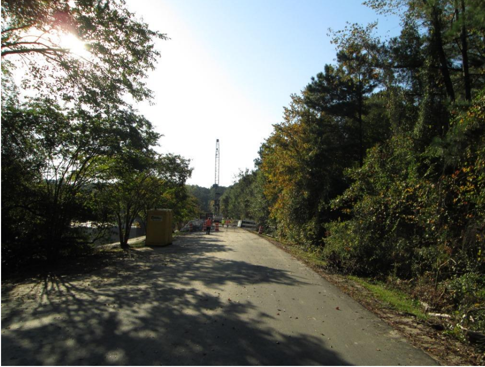
Photo 1: Roadway along embankment crest viewed from right embankment
