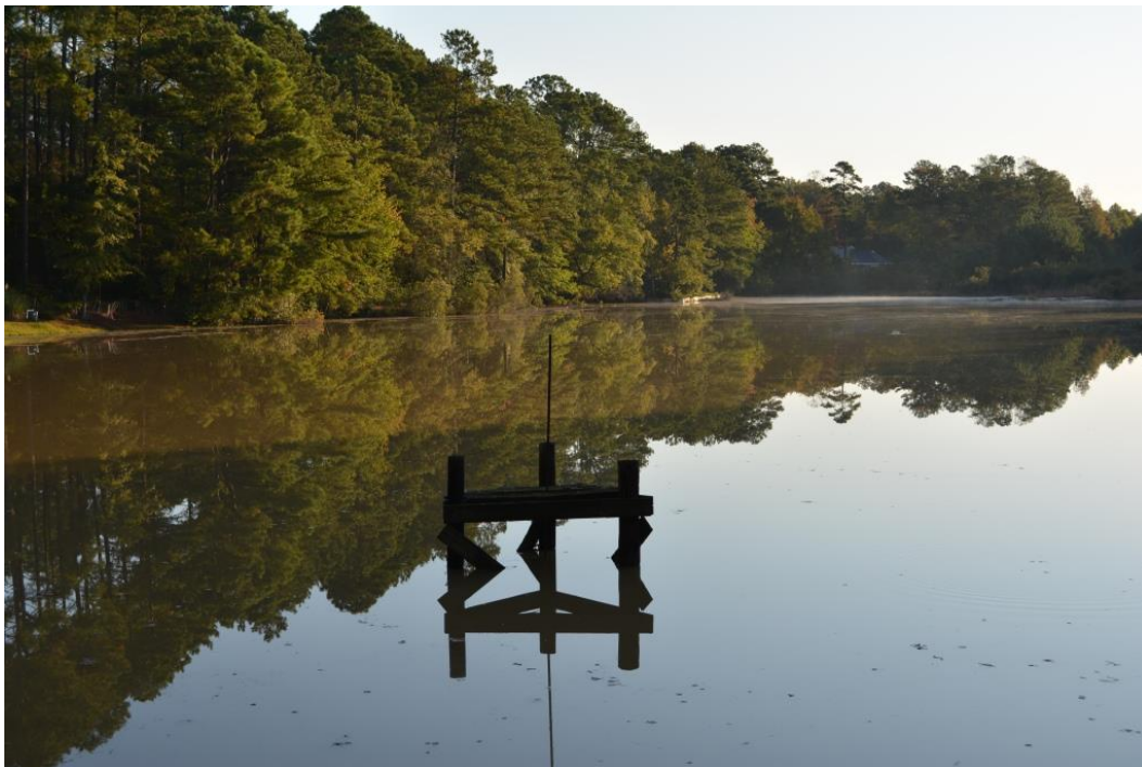
Photo 6: Service spillway intake platform
