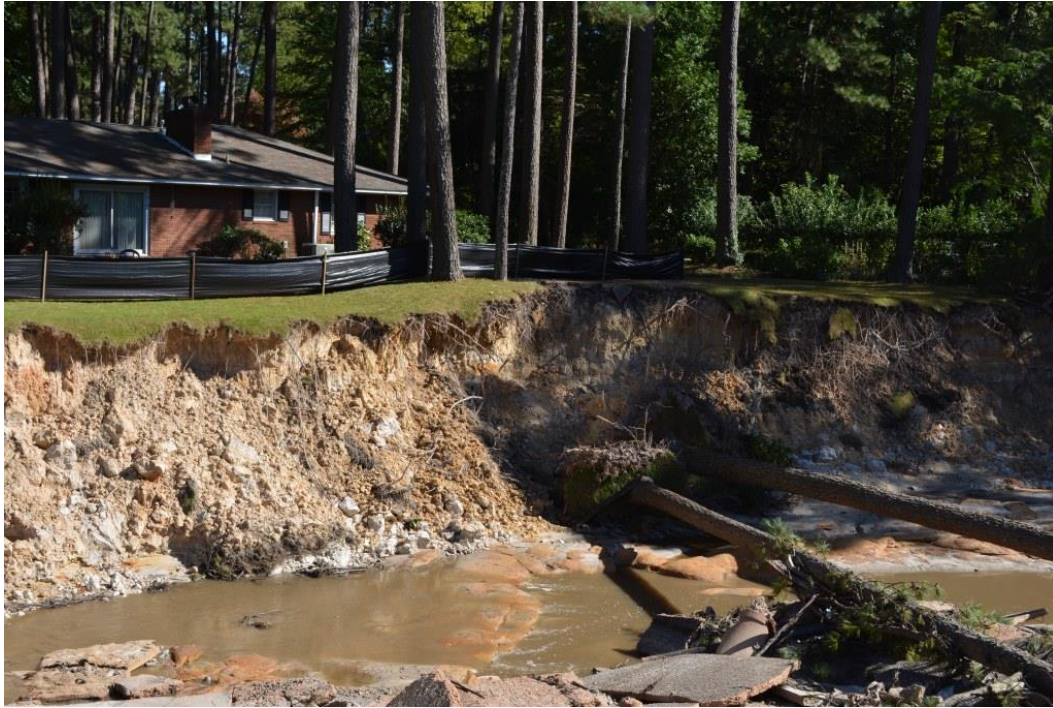
Photo 5: Erosion along the left side of the auxiliary spillway, looking downstream from the bridge
