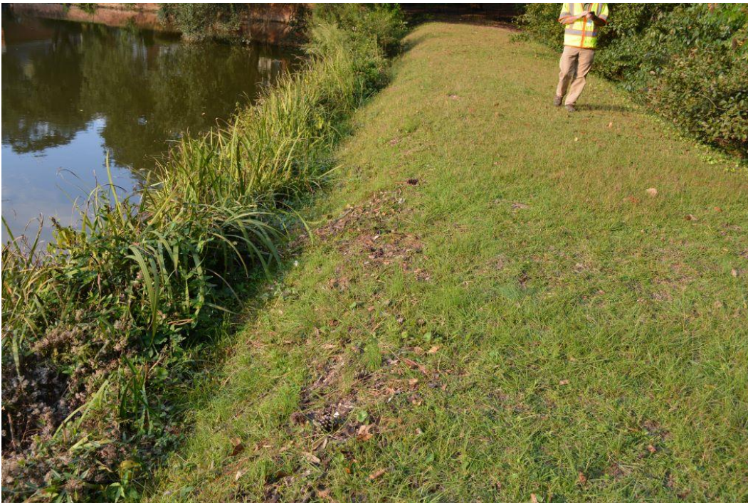
Photo 2: Upstream embankment slope and debris indicating peak flood level
