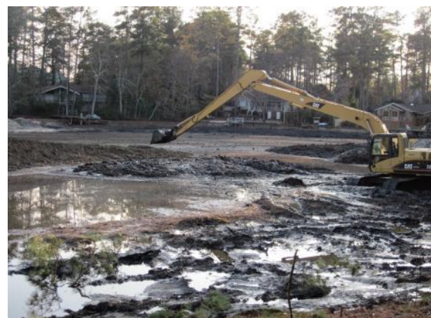
Removing sediment on Cary Lake
